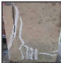
Figure6: Crack Pattern for Axial Load
