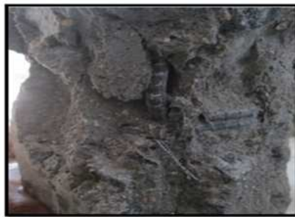
Figure 8: Crack Pattern for Biaxial Load
