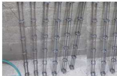
Figure 4: Reinforcement Cages 6mm DIA Bars Are Used As Ties
